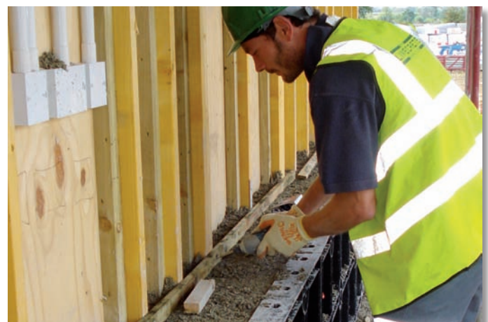
Pouring Tradical® Hemcrete® at Social Housing Development, Norfolk
