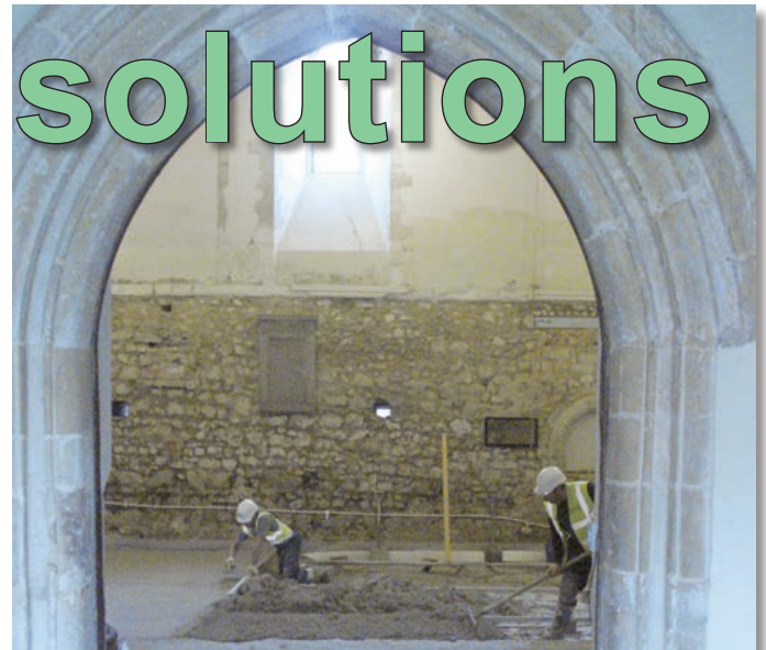
Placing the limecrete slab at St Thomas of Canterbury Church, Goring
