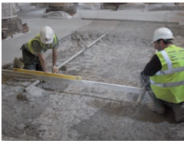
Screed rails at St Thomas of Canterbury Church, Goring
